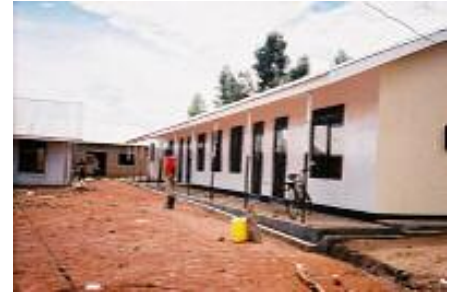
The new block just before moving in
